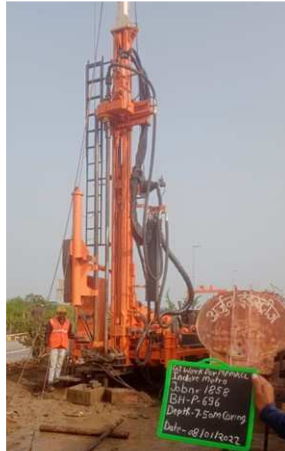
Performing Rock Drilling
