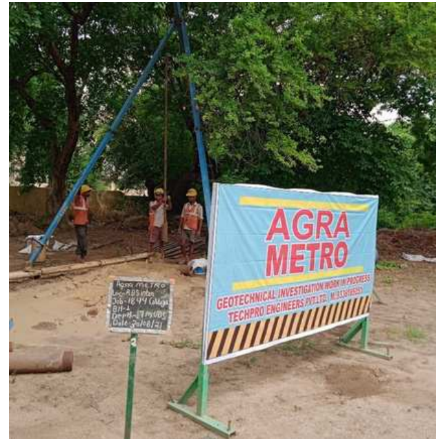
Extracting un-disturbed sample
