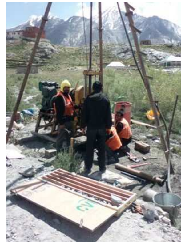
Performing Rock Drilling
