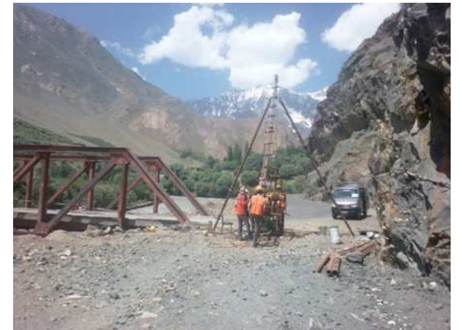
Performing Rock Drilling
